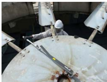
Pict. 14 Tighten torque bolt of hub plate.
