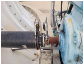
Pict. 8 Adjust drive shaft alignment after motor.
