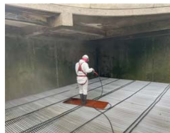
Pict. 7 Clean drift eliminator by high pressure water jet.
