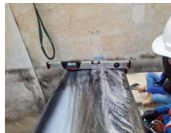
Pict. 18 Check fan blade pitch angle after tighten torque bolt.
