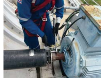
Pict. 10 Tighten torque bolt of drive shaft coupling motor.
