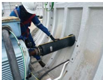
Pict. 13 Check distance between shaft ends after.
