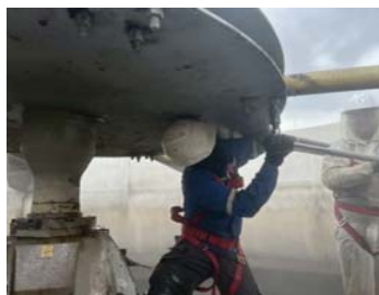
Pict. 15 Tighten torque bolt of fan blade.
