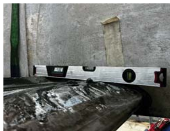
Pict. 7 Check fan blade pitch angle before tighten torque bolt.
