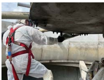
Pict. 15 Tighten torque bolt of fan blade.
