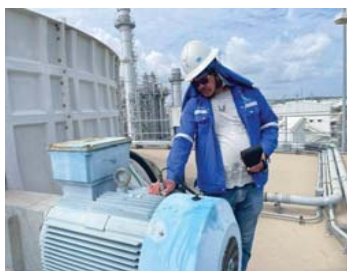
Pict. 23 Test run and vibration measurement.
