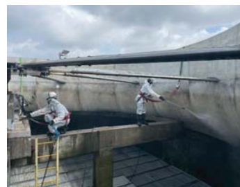
Pict. 6 Clean cooling tower by high pressure water jet.
