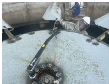
Pict. 14 Tighten torque bolt of hub plate.
